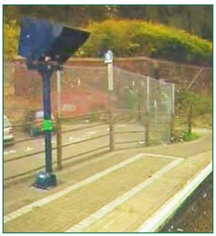
Figure 15: Eight-car monitor position in 2004. The head of the DOO monitor is now parallel to the platform edge (photograph courtesy of Network Rail)
