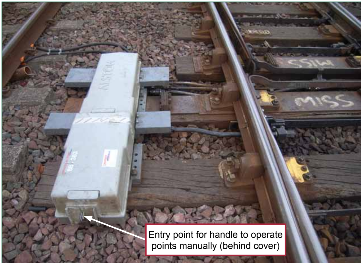
Figure 5: An HW2000 type point machine
