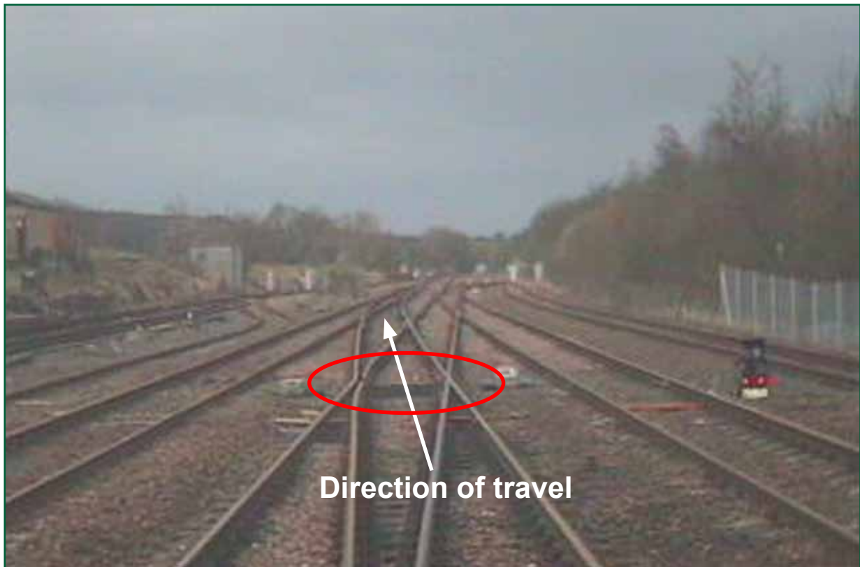
Figure 4: Forward view of Greenhill Upper Junction as train 2N50 approached showing the position of 125C point ends (normal) and 125B point ends (reverse)
