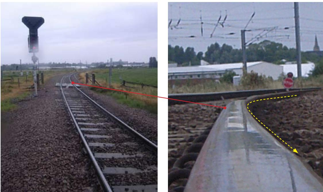
*Figures 8 (left) showing view of track towards Ely with right high rail on left and low left rail on right. Figure 9 (right) view of track towards Ely showing low left rail (foreground) and high right rail (background) at the point of derailment*
