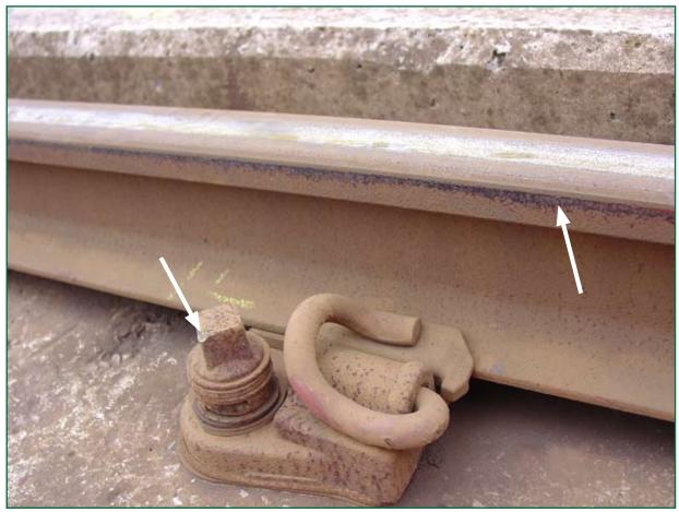
Figure 5: Cess side rail showing marks left by wheel (arrowed)
