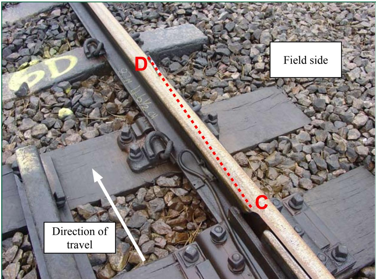
Figure 11: Photograph of adjustment switches showing point of impact with the machined notch (C) and derailment mark indicated by the position of the pen on rail head (D) where right hand wheel landed after being in free flight for 700 mm (grinding marks are visible on the rail head, showing light corrosion following overnight rain).
