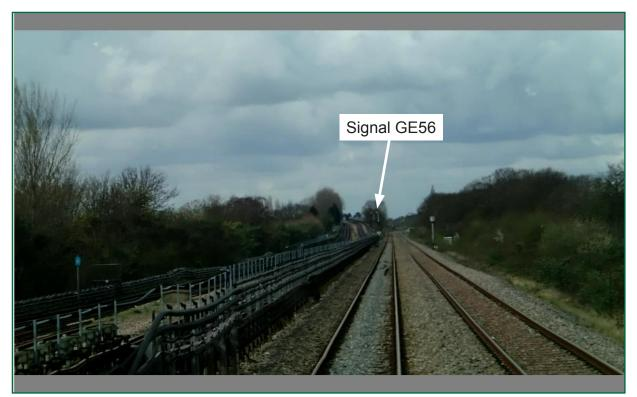
Figure 10: View of signal GE56 at clear, from 650 yards (594 metres) away
