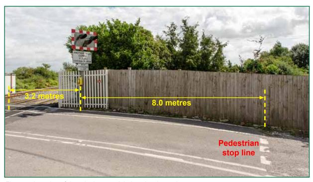
Figure 7: Location of the telephone at Athelney level crossing
