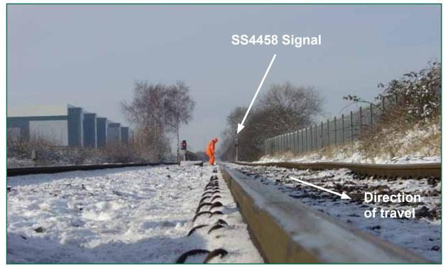
Figure 9: Cyclic top on the up Chellaston just before the point of derailment on the day following the derailment
