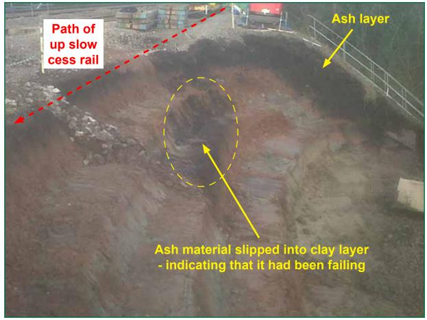
Figure 12: The embankment after being dug out (photograph courtesy of Network Rail)
