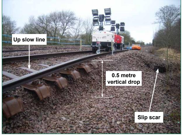
Figure 8: Scars showing embankment slip
