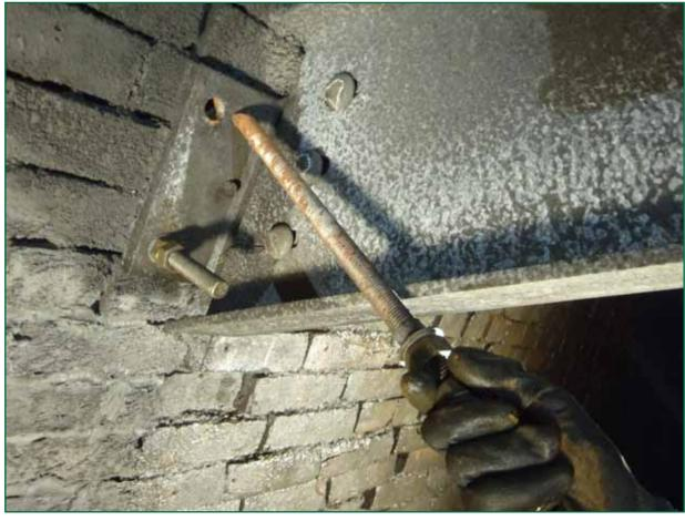
Figure 12: Loose stud outside incident area removed by hand during inspection on 23 September 2011 (photograph courtesy of Amey)
