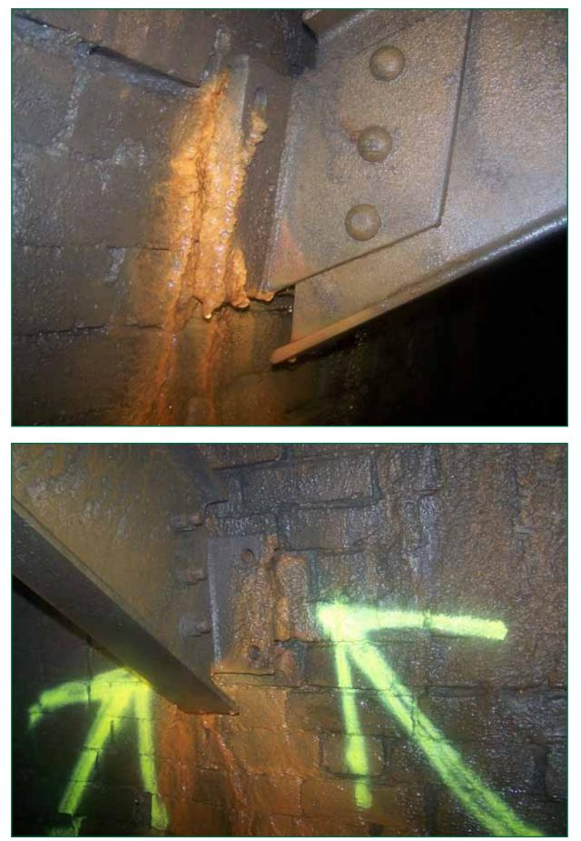
Figures 18 and 19: Missing studs at chainage 34 in November 2008 (photographs courtesy of Network Rail)
