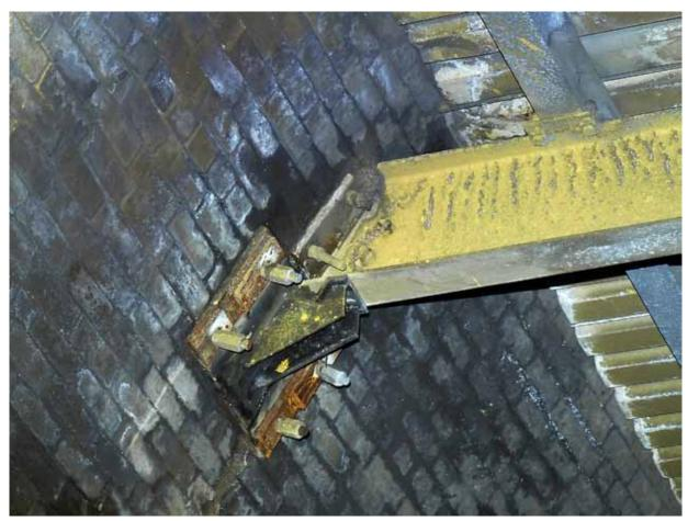
Figure 24: Transverse beam end after fitting of additional support bracket post-incident
