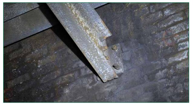
Figure 8: Transverse beam (as designed) supported by two studs on each side of the beam end
