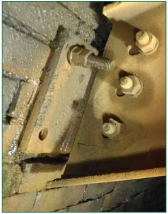
Figure 11: Bracket with lower stud found missing (photograph courtesy of Amey)
