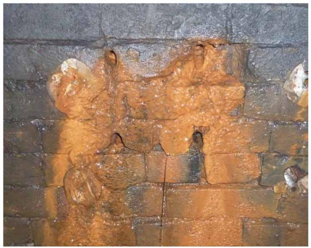
Figure 16: Former position of transverse beam 16 (up side) - note running water
