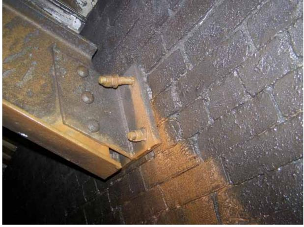
Figure 20: Loose stud sent to SME1 in March 2009 (photograph courtesy of Network Rail)
