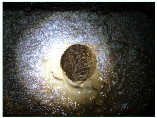
Figure 13: Hole in brickwork from which studs had fallen, showing thread pattern imprint
