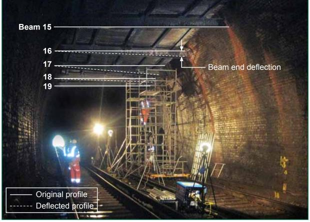
Figure 9: View of deflected structure on 23 September 2011 (photograph courtesy of ORR)
