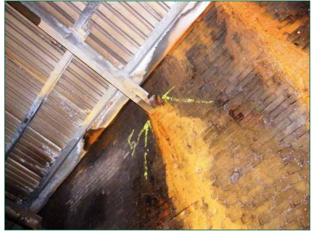
Figure 21: Missing studs at chainage 34 (June 2011) (photograph courtesy of Amey)
