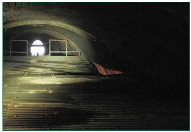
*Figure 10: View of deflected structure from above, looking towards the south end of the tunnel, showing the twisted deck on the right-hand side (photograph courtesy of Amey)*
