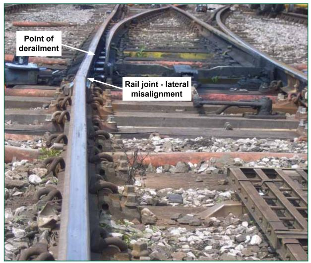
Figure 8: Track lateral alignment approaching No. 75 points
