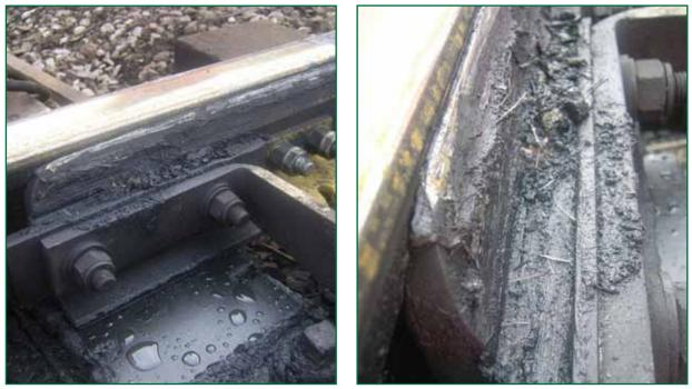
Figure 9: Left-hand switch rail at No.75 points immediately after derailment
