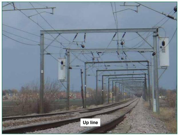
Figure 24: Portal structures immediately before mast C119/04 (courtesy of First Capital Connect)
