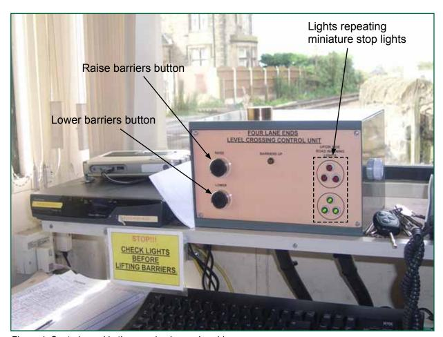
Figure 4: Control panel in the crossing keeper's cabin
