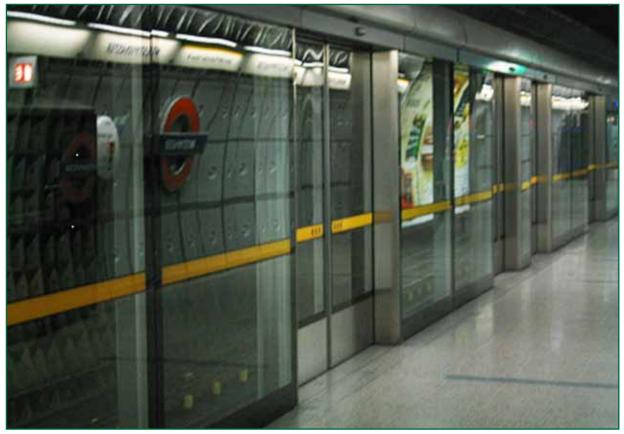
Figure 18: Platform edge doors on London Underground (Courtesy of Transport for London)
