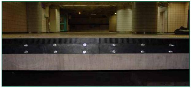
Figure 27: Gap filler bolted to the platform edge
