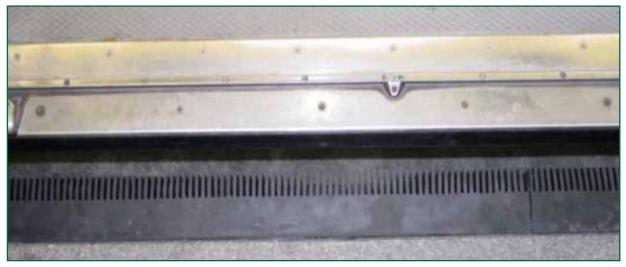
Figure 28: The platform edge after fitting gap filler
