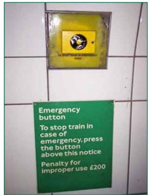
Figure 17: Platform mounted emergency stop button
