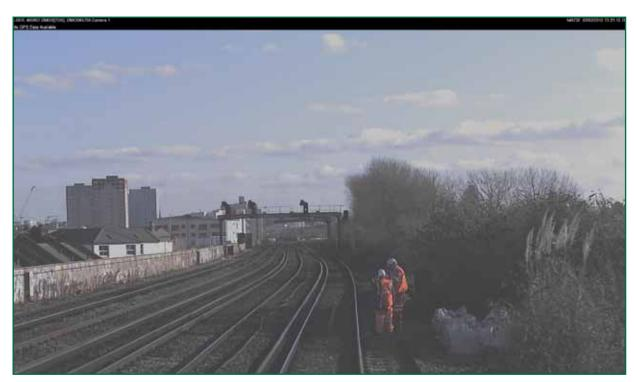
Figure 2: Forward facing CCTV image from train 2N36. The lookout has his back to the approaching train. The COSS is positioned to the right of the lookout. The supervisor is just beyond the COSS and cannot be seen in this image.
