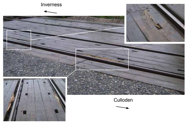
Figure 12: Detailed pictures of damage to Drumrosach RRAP
