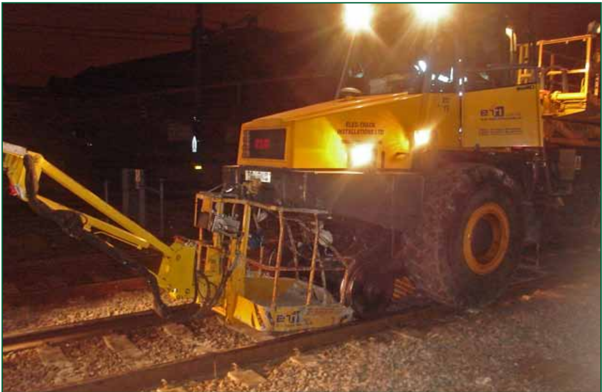
Figure 7: Damage as result of the TD-18 RRV colliding with the Basket 14 RRV (Photograph courtesy of Mouchel Rail Ltd)
