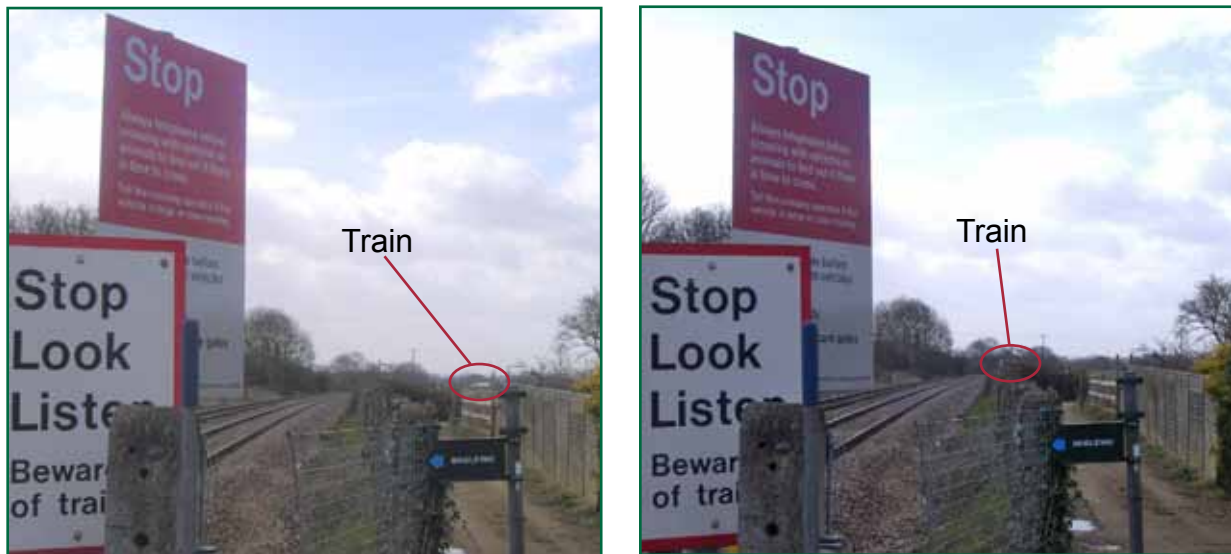
Figures 5 & 6: Train approaching on the down line, viewed from the down side of crossing outside of the wicket gate. The train is visible in the distance (Figure 5), but becomes hidden by vegetation as it approaches the crossing (Figure 6)
