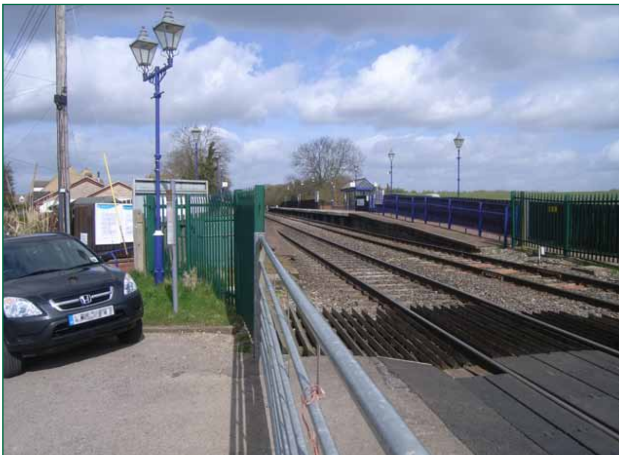
Figure 3: Visibility from the down side of the crossing to the north, photographed from outside of the railway boundary
