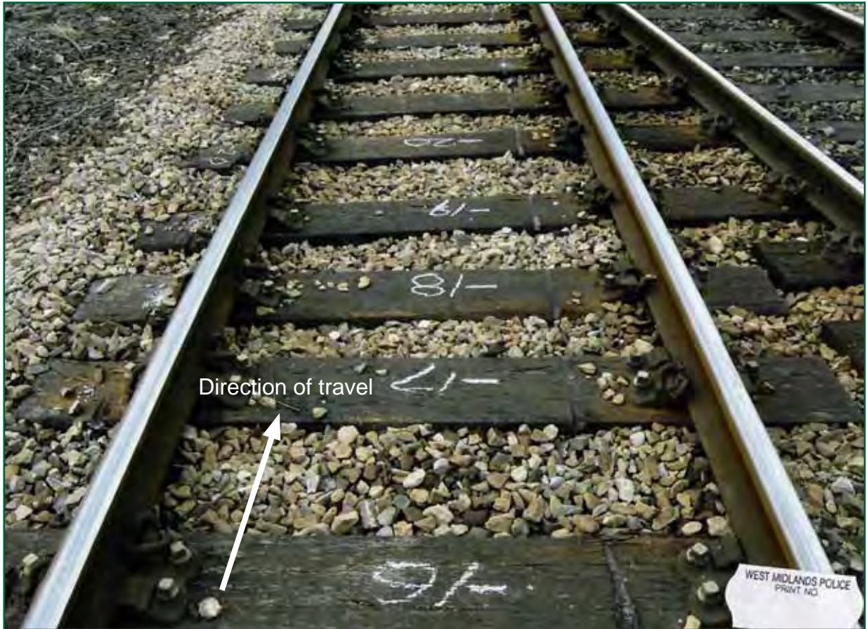
Figure 7: Damage marks (photograph courtesy of West Midlands Police)
