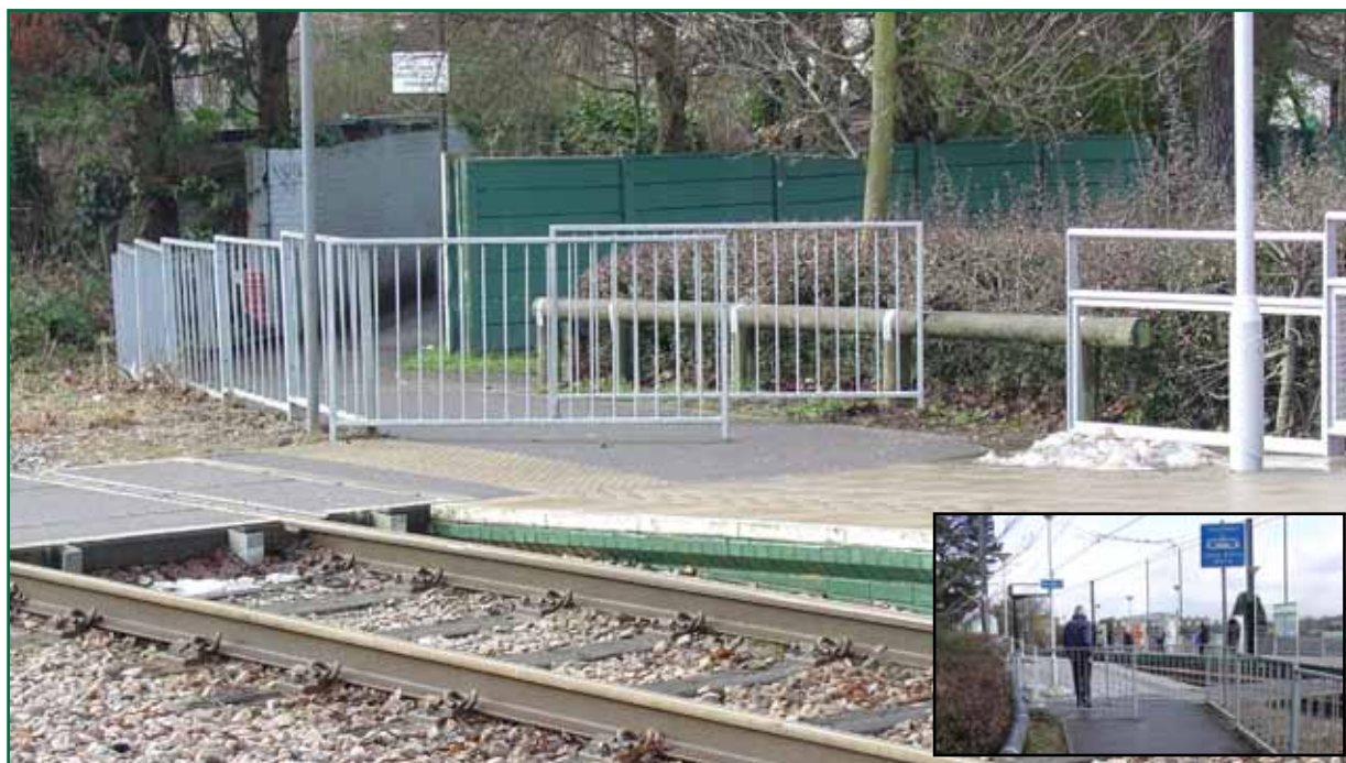
Figure 7: Chicane installed at Arena tram stop
