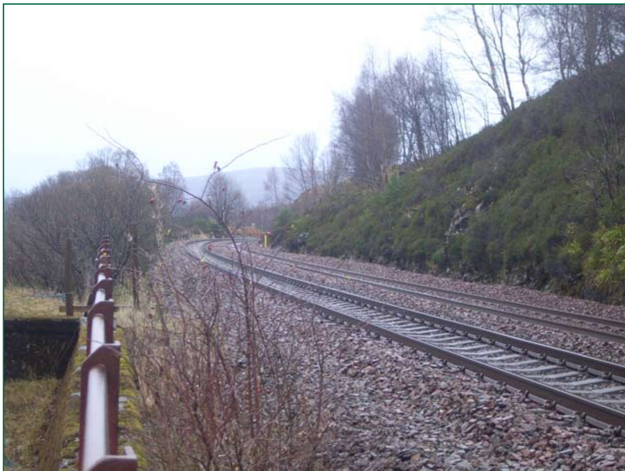
Figure 7: View towards the rock drilling site from the approximate location of the vegetation chipping site
