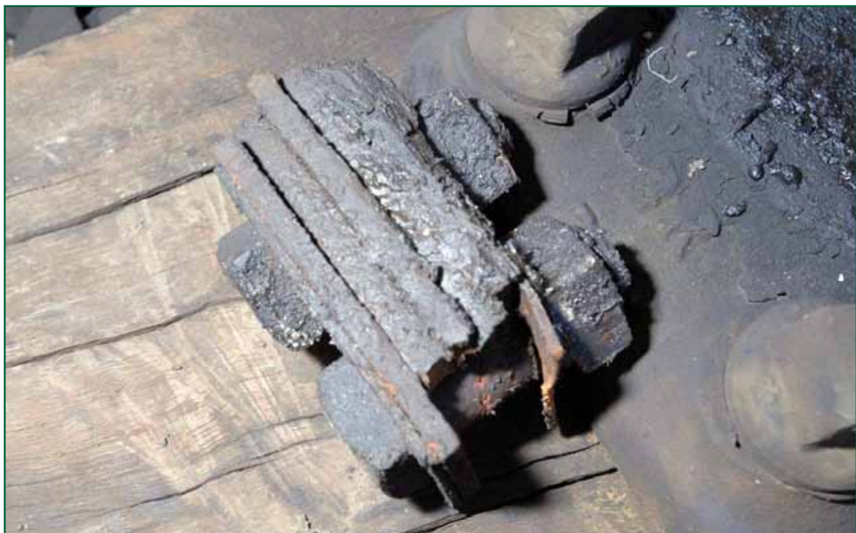
Figure 21: The third permanent way stretcher bar swan neck insulation assembly
