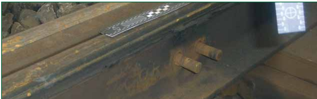
Figure 17: Right-hand switch rail at second permanent way stretcher bar position
