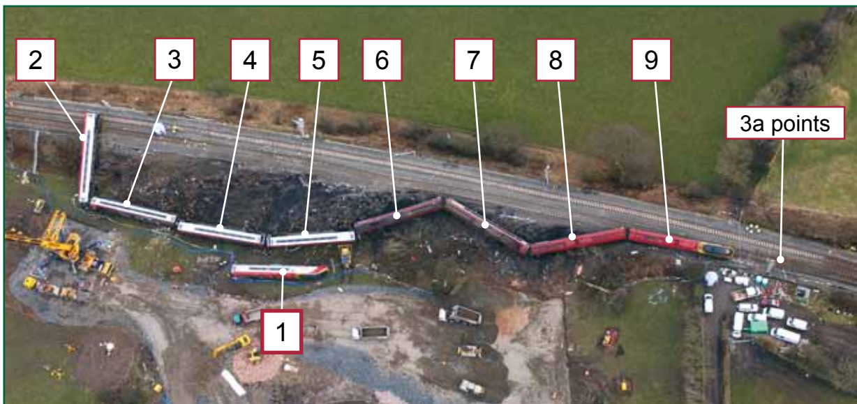
Figure 2: Aerial view of derailed train
