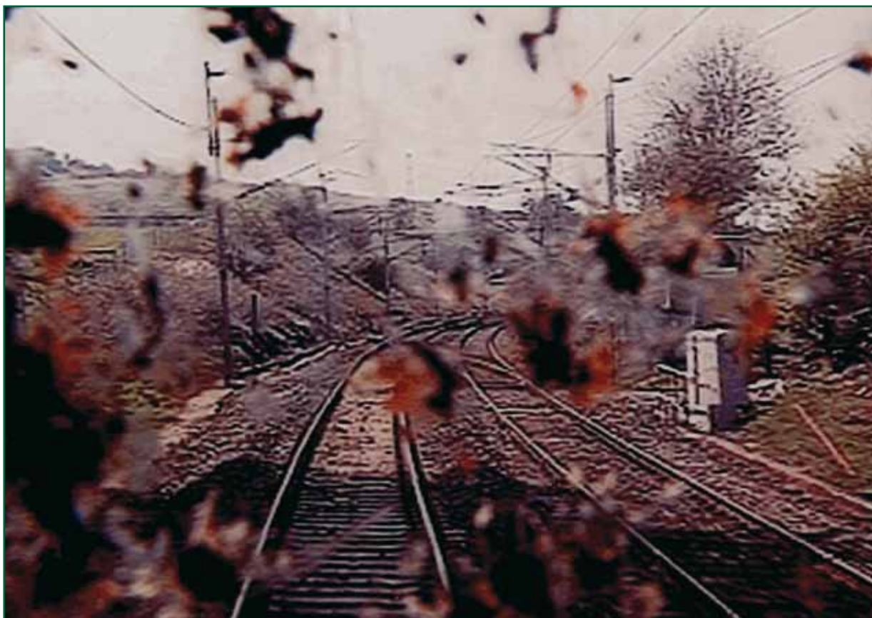
Figure 47: Approach to Lambrigg viewed from the up line in May 2006. Scrap rail behind location cabinet is visible
