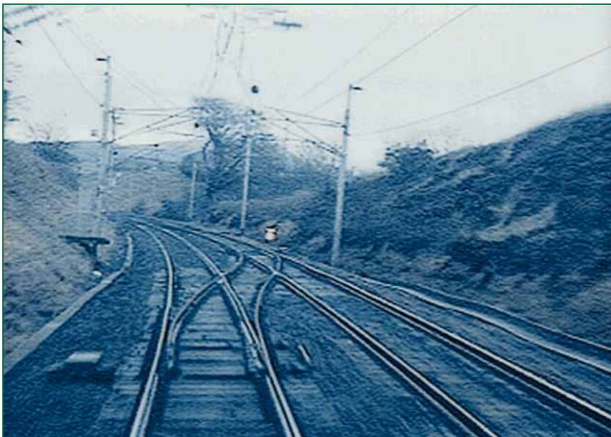
Figure 48: Points 2B viewed from the front of the NMT on 10 January 2007
