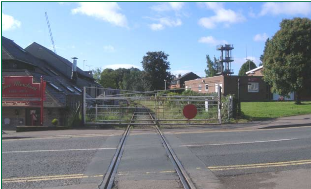
Figure 3: Lydney town crossing looking south
