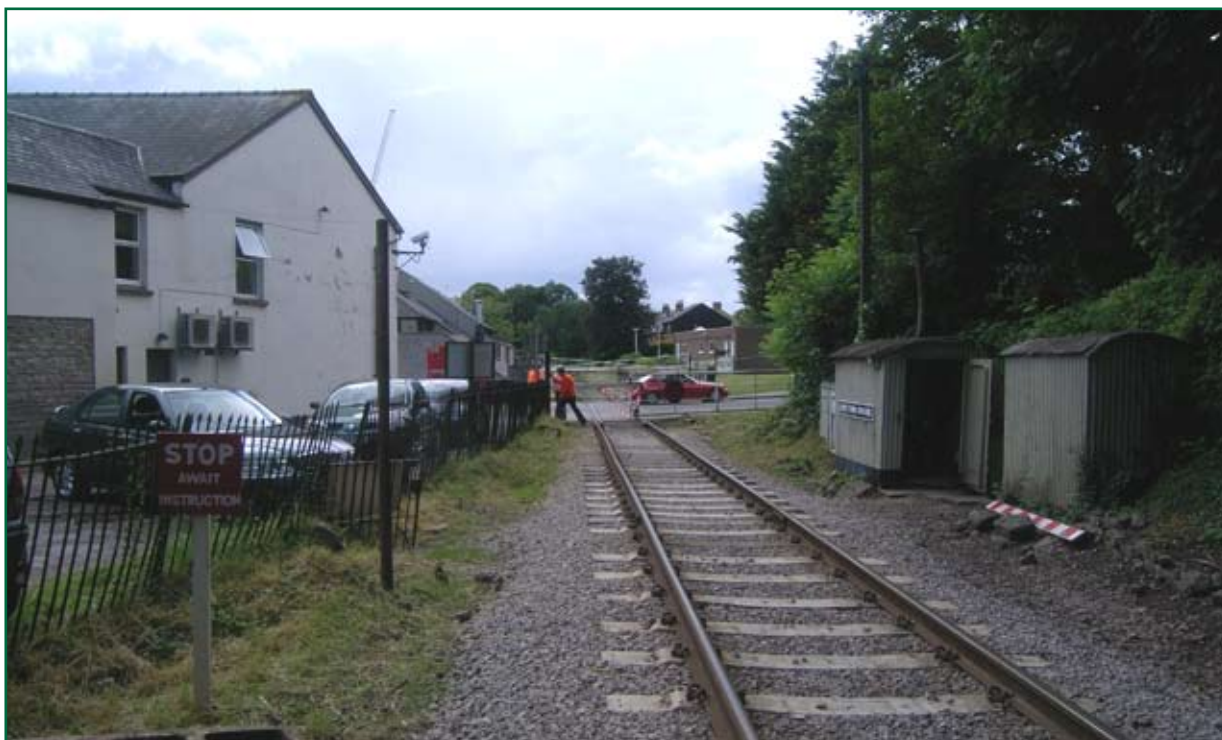
Figure 8: Approach to Lydney Town crossing, showing 'Stop' board
