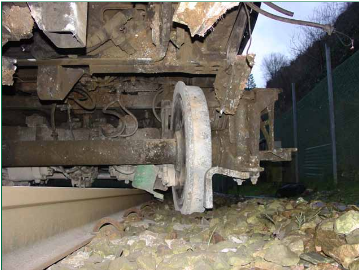
Figure 13: Damage to the front bogie of the train
