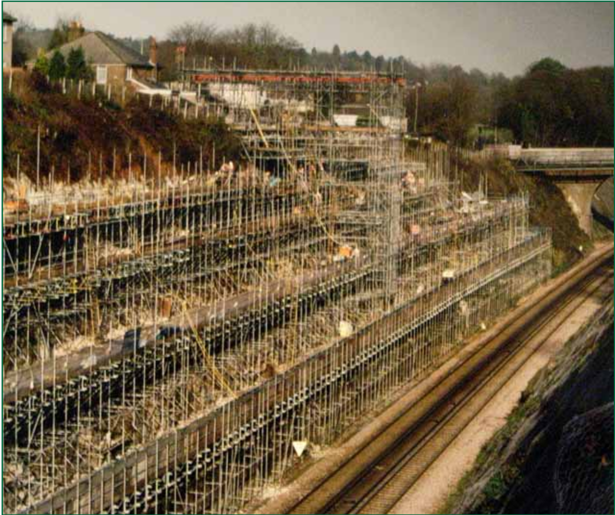
Figure 15: Photograph showing the stabilisation works of 2001 - 3 (courtesy of Network Rail)
