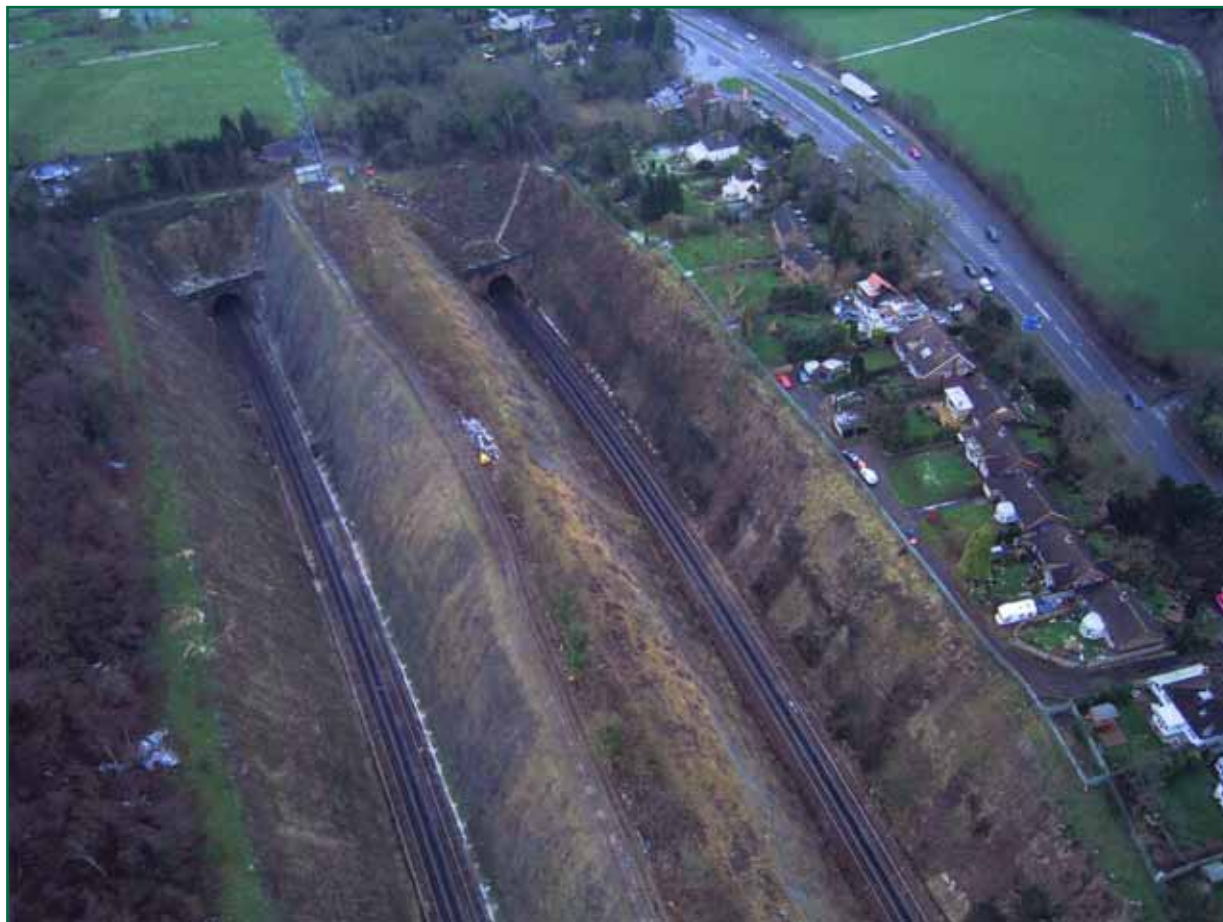
Figure 4: Aerial photograph of the two lines at Merstham in 2007. The Redhill slow lines are on the right and the Quarry fast lines on the left (courtesy of Network Rail)
