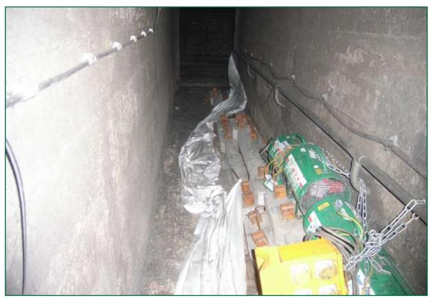
*Figure 9: Equipment stored in the cross passage as found immediately following the derailment and viewed looking towards the westbound track*
