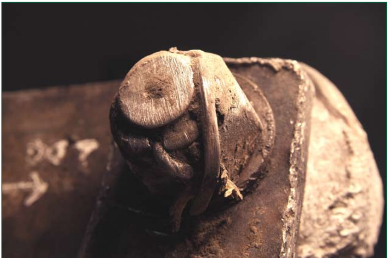
Figure 13: Lower torque arm fixing bolt with post incident damaged castle nut and split pin. Wooden debris from a cattle grid stake is also visible
