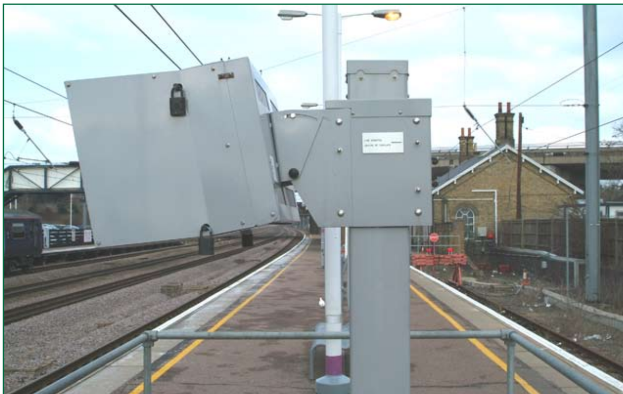
Figure 10: Side view of the four-car DOO monitor bank
