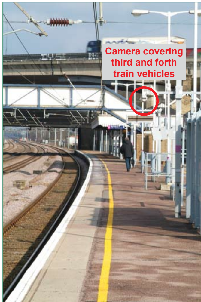
Figure 16: Location of CCTV camera covering last two vehicles
