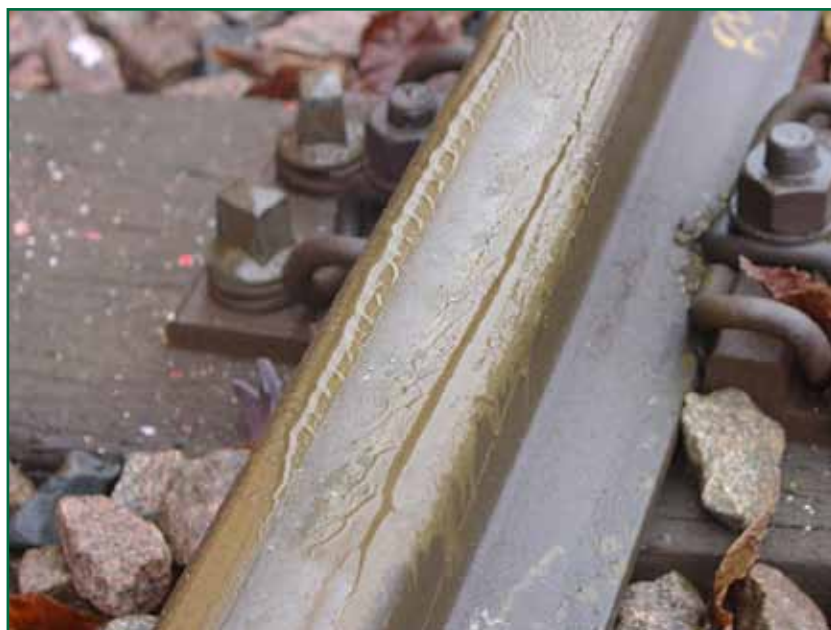
Figure 5: Rail condition in the vicinity of KHD02 signal
