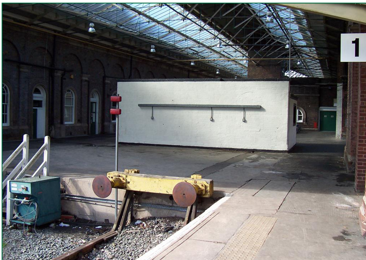
Figure 5: Buffer stop in platform 1 prior to accident and before installation of a glass screen (courtesy of Network Rail)
