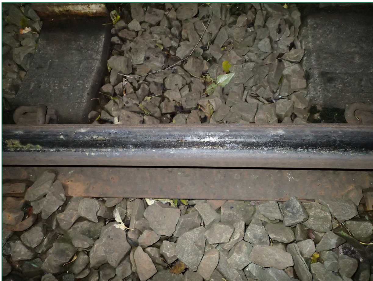
Figure 9: Rail contaminated with leaf material at AWS magnet for signal CR27
