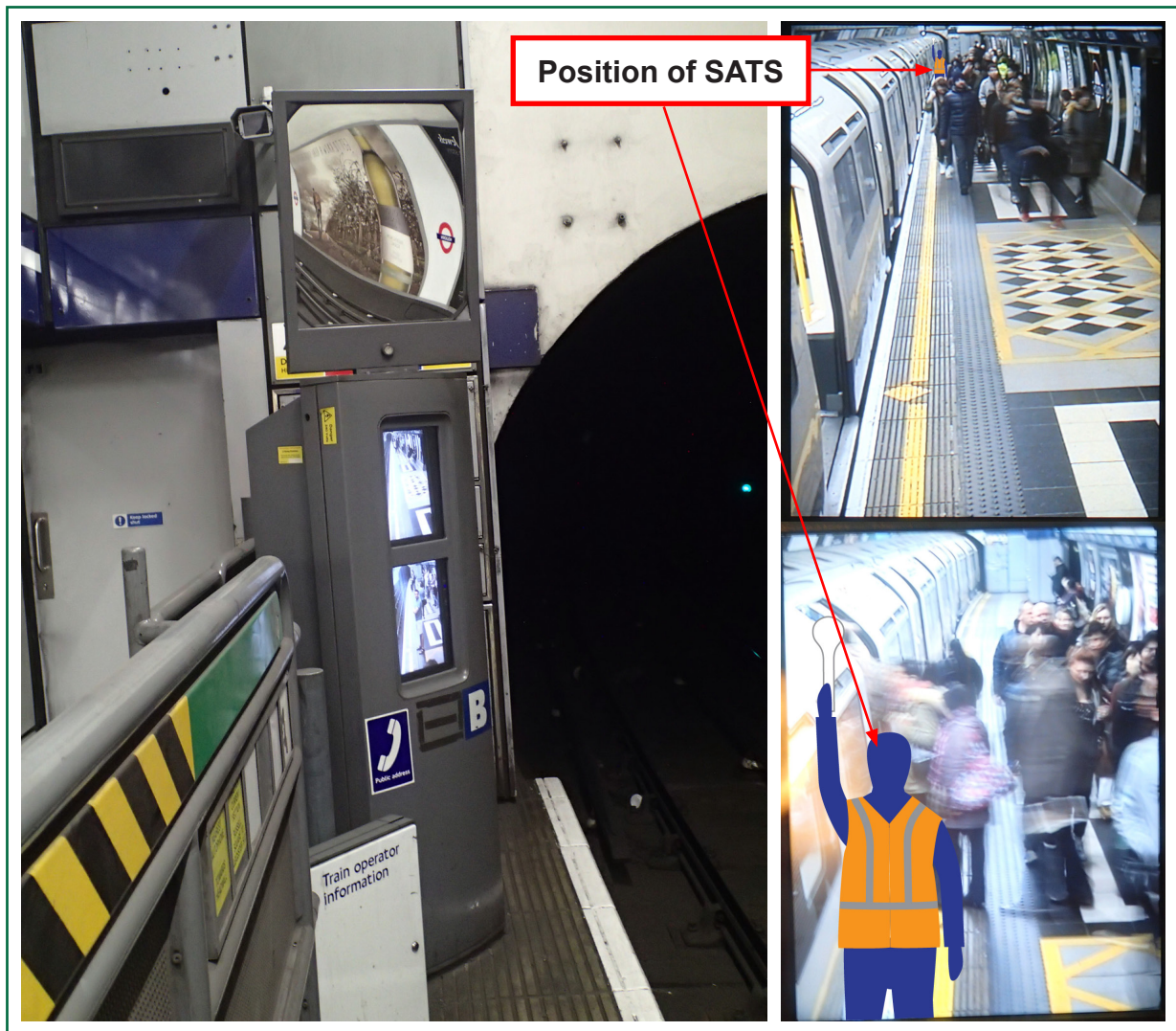
Figure 6: Train despatch mirror and CCTV monitors on Holborn westbound Piccadilly line platform, showing position of SATS as he would have appeared on both monitors
