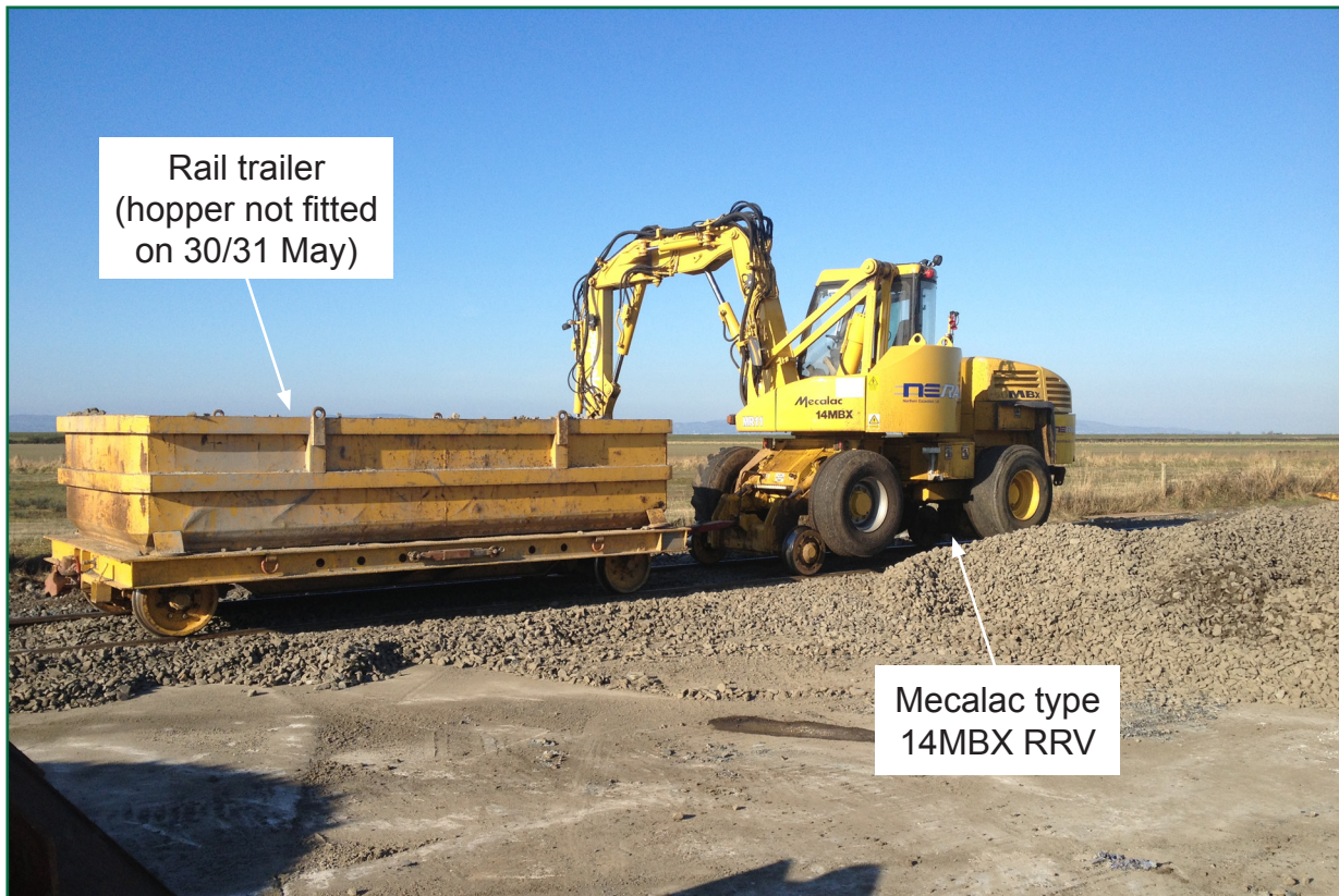
Figure 6: A Mecalac type 14MBX RRV and rail trailer – note that the trailer would not have been loaded with a hopper on 30/31 May 2013 (image courtesy of Northern Excavators Ltd)
