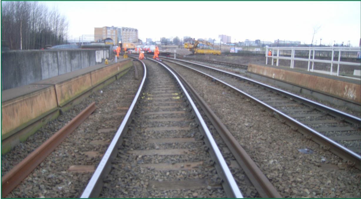
Figure 4: The track on the Down Bolton line, looking from bridge 130B towards the derailment site
