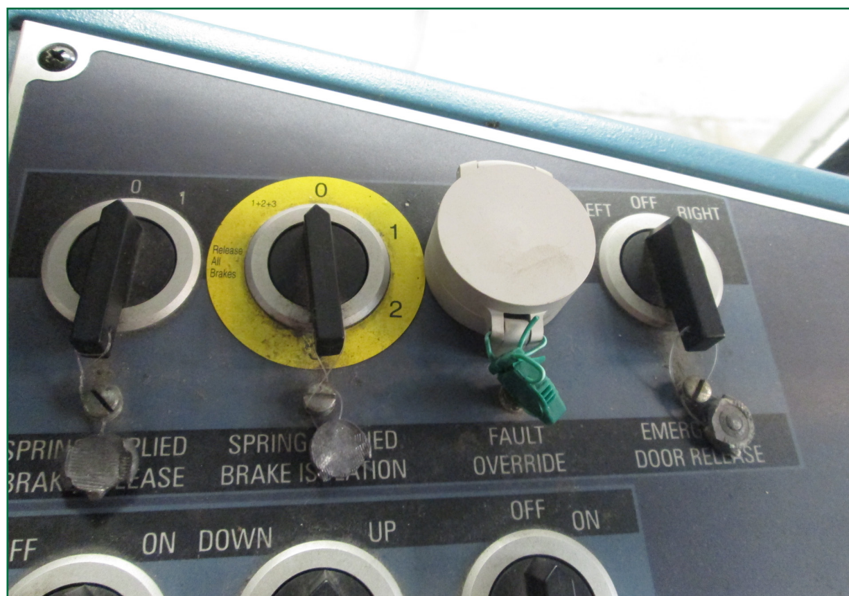
Figure 9: Bombardier key switch modification for fault override.
