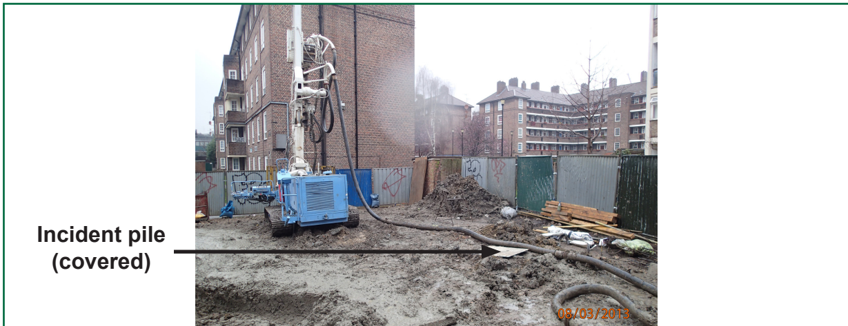
Figure 3: Piling rig on site at East Road
