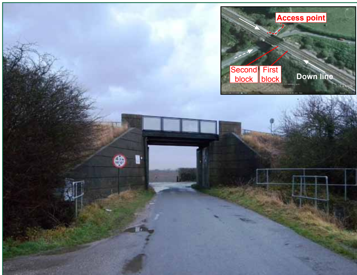
Figure 3: Sykes Lane underbridge and (inset) Google Earth image showing locations of access point and areas of work for the first and second line blockage
