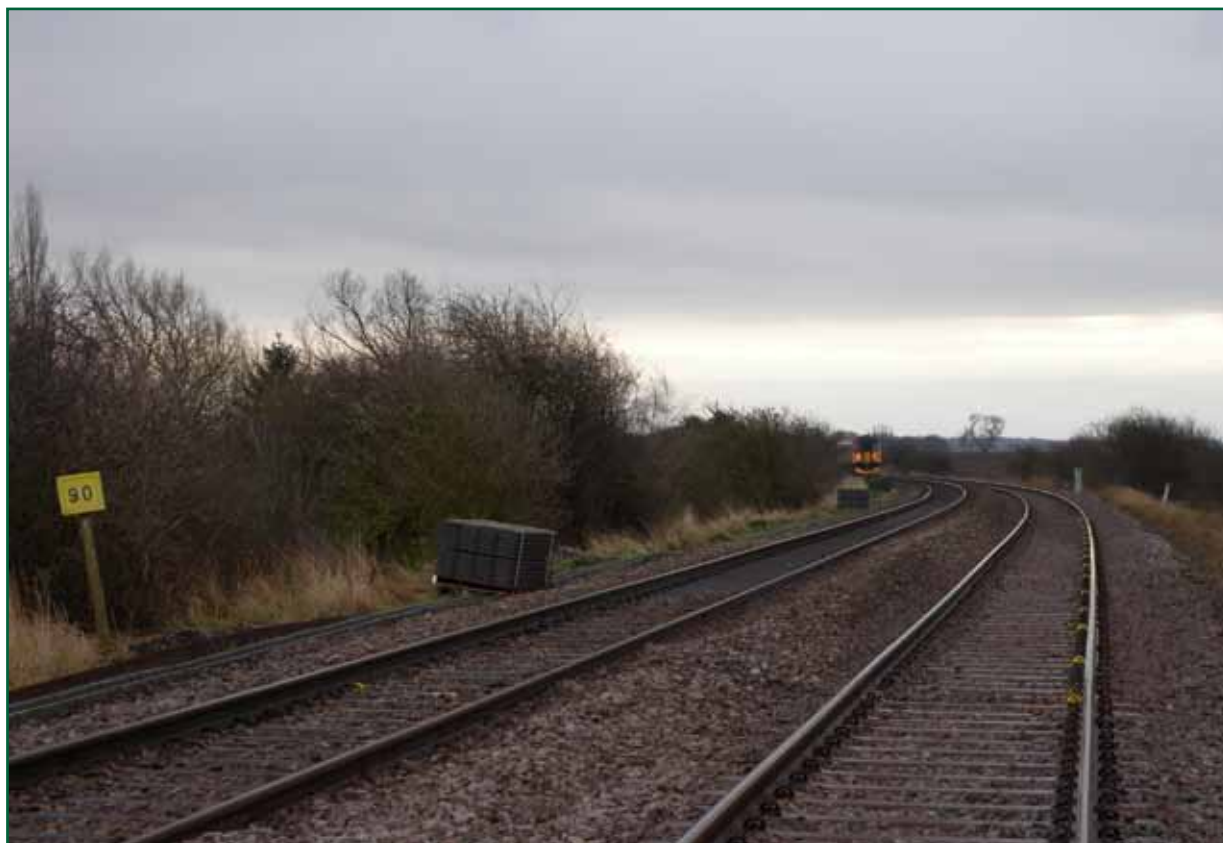
Figure 5: The down line at the scene of the accident, looking in the opposite direction to figure 4, showing the available view of down trains
