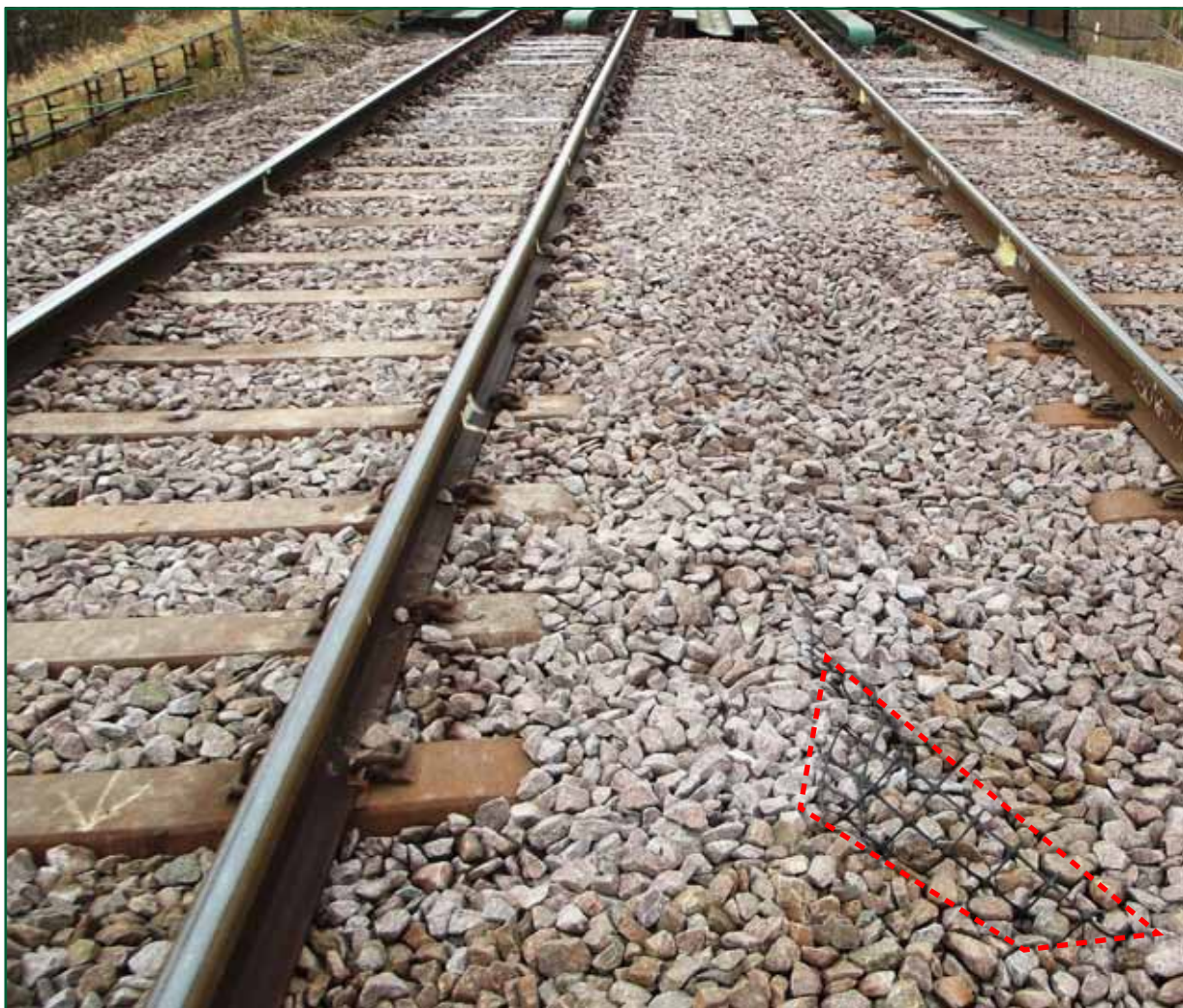
Figure 18: The geomesh at the site of the accident
