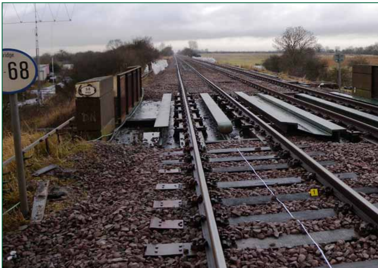
Figure 4: The scene of the accident, looking along the down line, showing the available view of trains approaching on the up line
