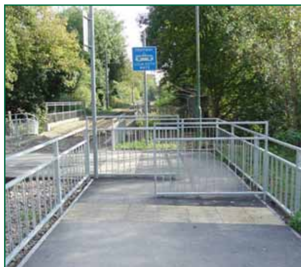
Figures 7a and 7b: Changes to the chicane at Morden Hall Park footpath crossing, London Tramlink
