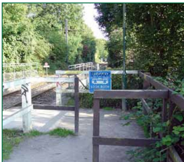
Figures 7a and 7b: Changes to the chicane at Morden Hall Park footpath crossing, London Tramlink
