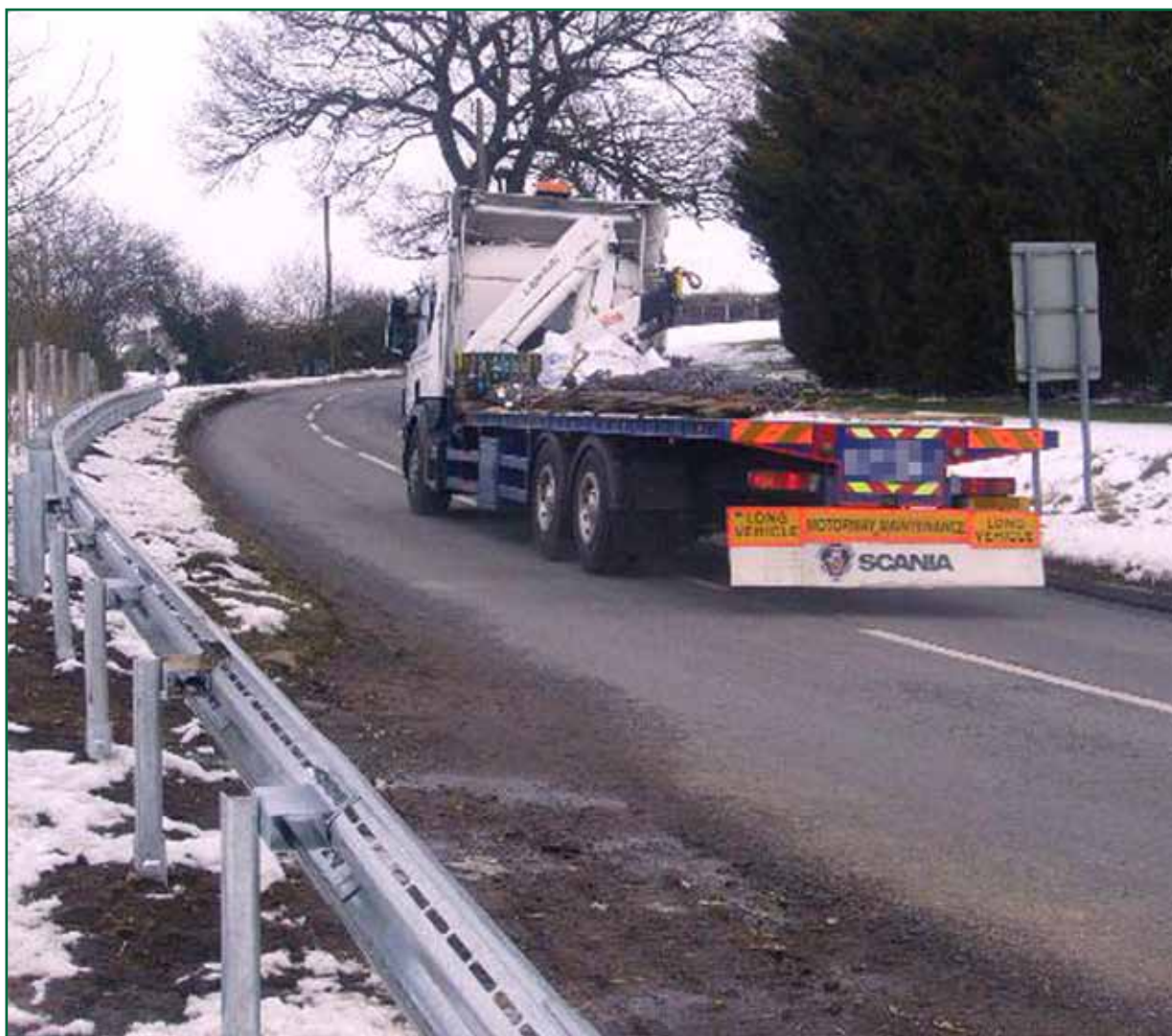
Figure 12: Image of a large goods vehicle negotiating the right-hand bend after the installation of the safety barrier (Feb 2012)
