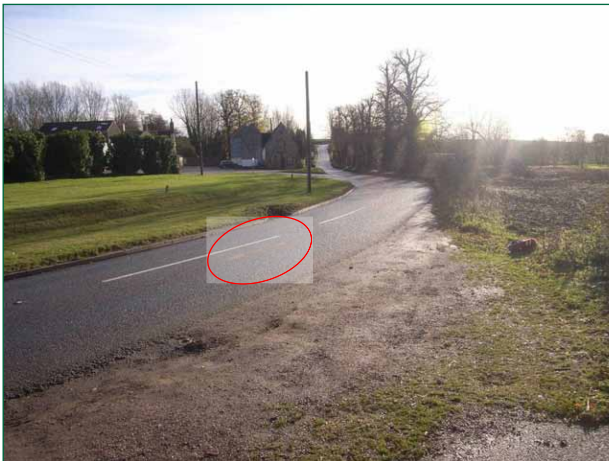
Figure 8: Image of the accident scene the following day (01/12/11) showing area of contamination (circled in red) on the road
