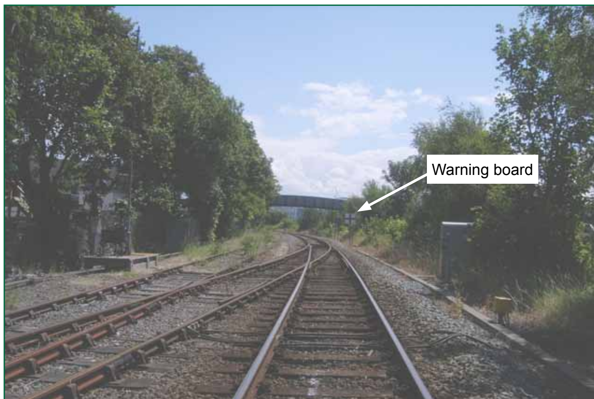
Figure 9: Warning board - as seen by an approaching train driver after leaving Aberystwyth station
