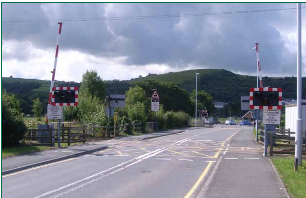
Figure 3: Llanbadarn ABCL crossing looking south along A4120 (with the Vale of Rheidol Railway AOCL crossing in the background)
