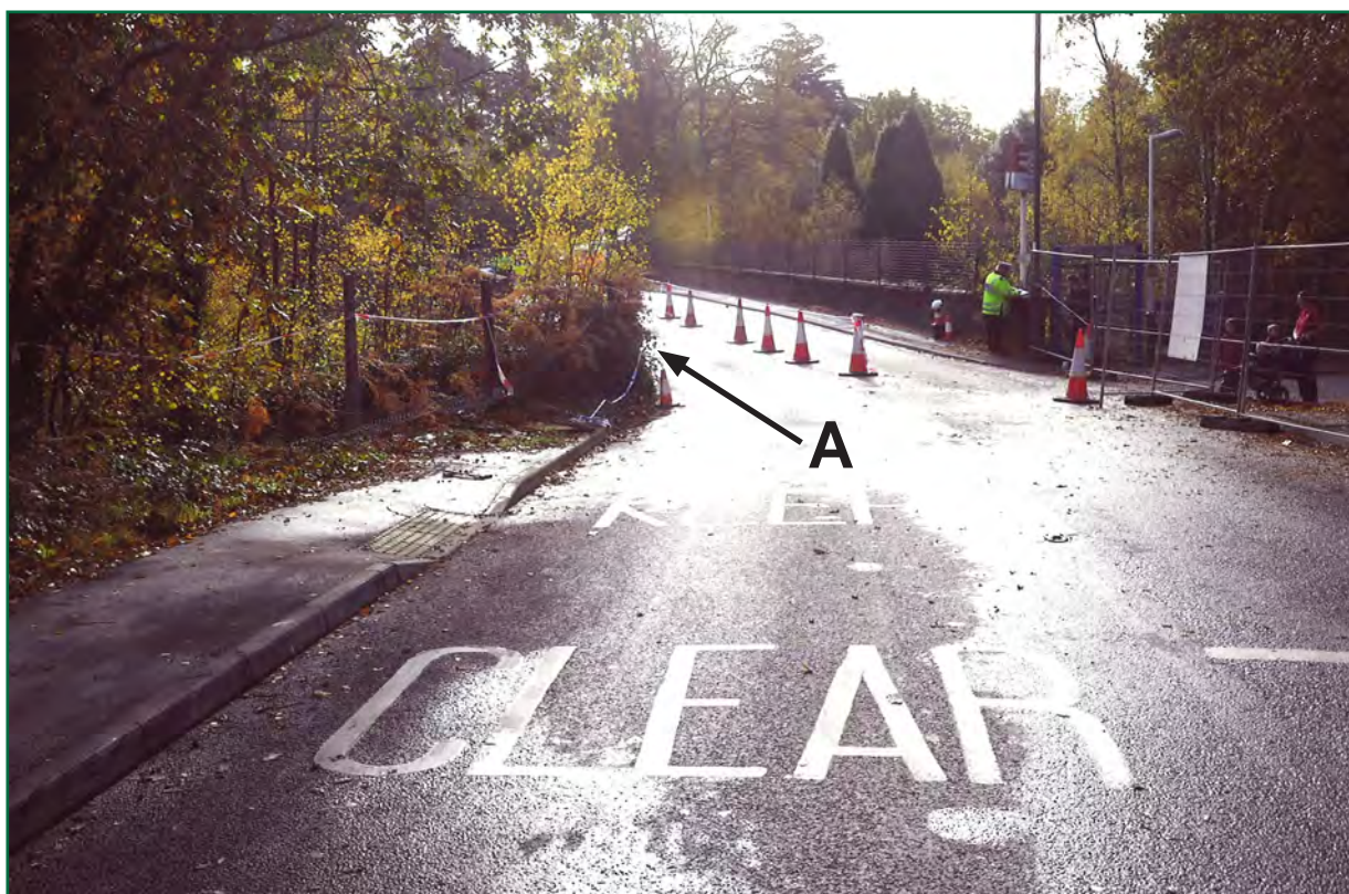
Figure 2: View of approach to bridge 11 for southbound traffic showing left-hand bend. The parapet end struck by the lorry is hidden by vegetation, and is marked 'A' (photograph courtesy of Surrey Police)
