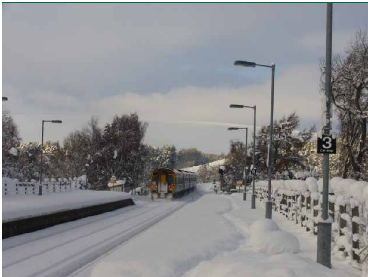
Figure 3: View towards the north end of Carrbridge station on 2 January 2010 (image courtesy of Roy Brown)
