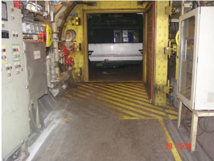
Figure 40: View of the amenity coach from the service tunnel through cross-passage 4898 (showing the window through which the majority of the passengers left)
