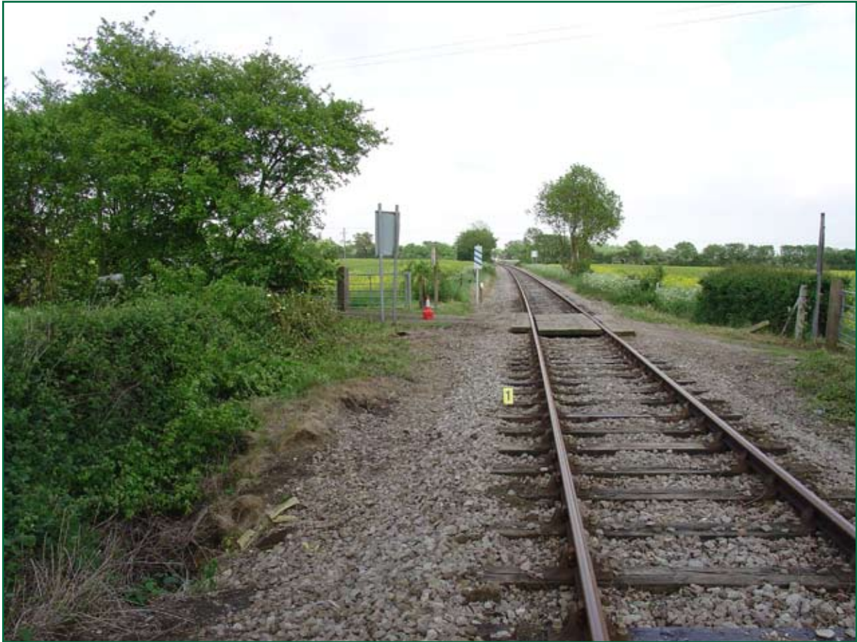
Figure 3: Bratts Blackhouse No 1 UWC as seen by trains travelling from Saxmundham to Sizewell (20 m from crossing). The cone is approximately 3 m from the nearest rail.
