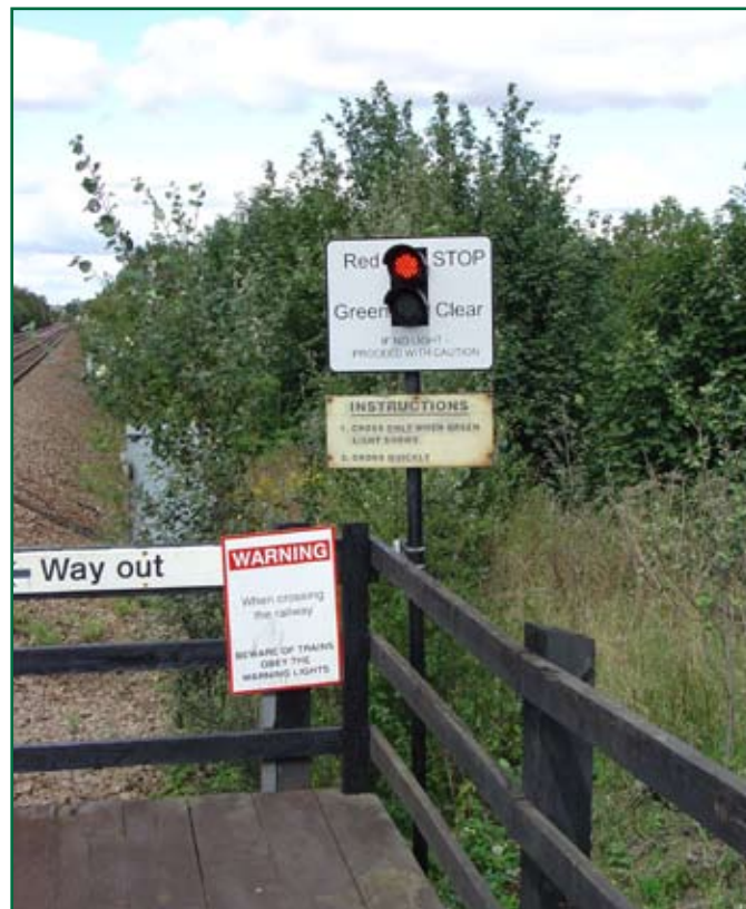
Figure 15: Modern pedestrian stop lights at Bolton-on-Dearne station
