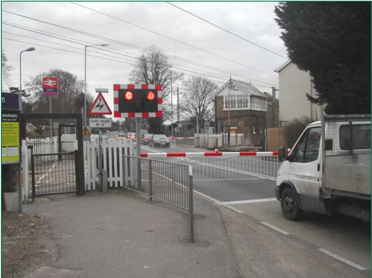
Figure 3: Example of SPC-GL (Foxton)
