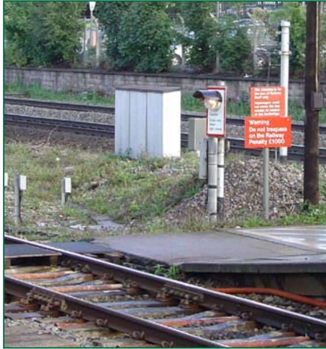
Figure 2: Typical example of a barrow crossing (Slough)
