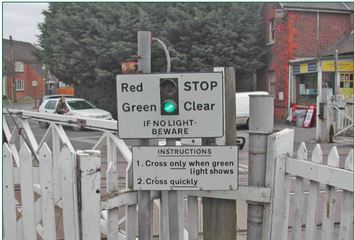
Figure 21: Upside miniature stop lights at Elsenham
