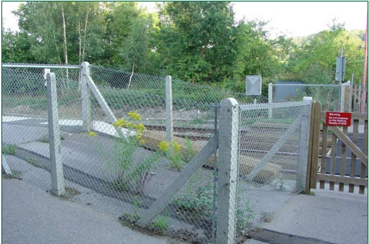
Figure 12: Fencing installed at Gomshall to direct passengers
