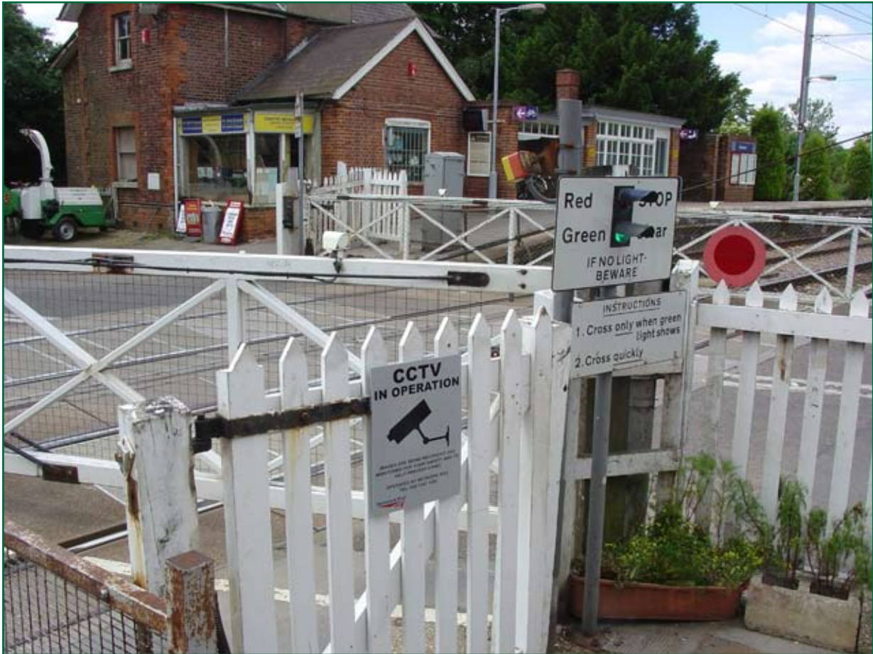
Figure 18: View of crossing signage and miniature stop lights on approach to Upside pedestrian gate from platform 1
