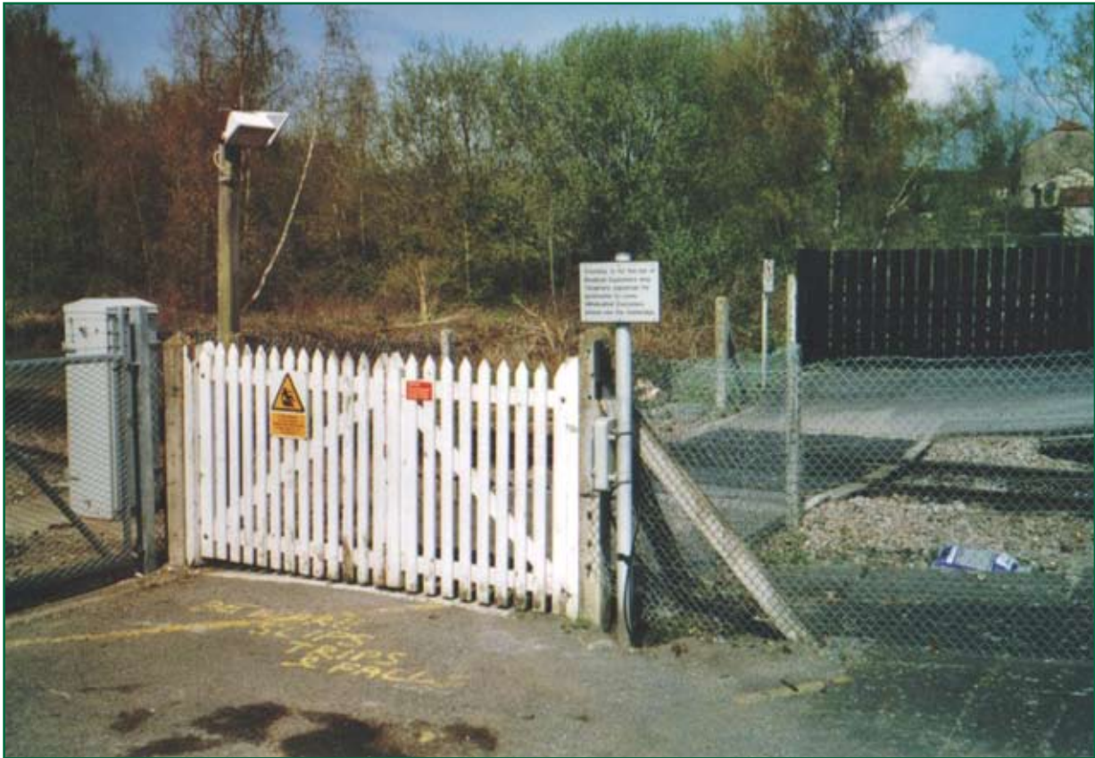
Figure 16: Pedestrian foot crossing retained for use by disabled passengers under the supervision of railway staff (Templecombe)
