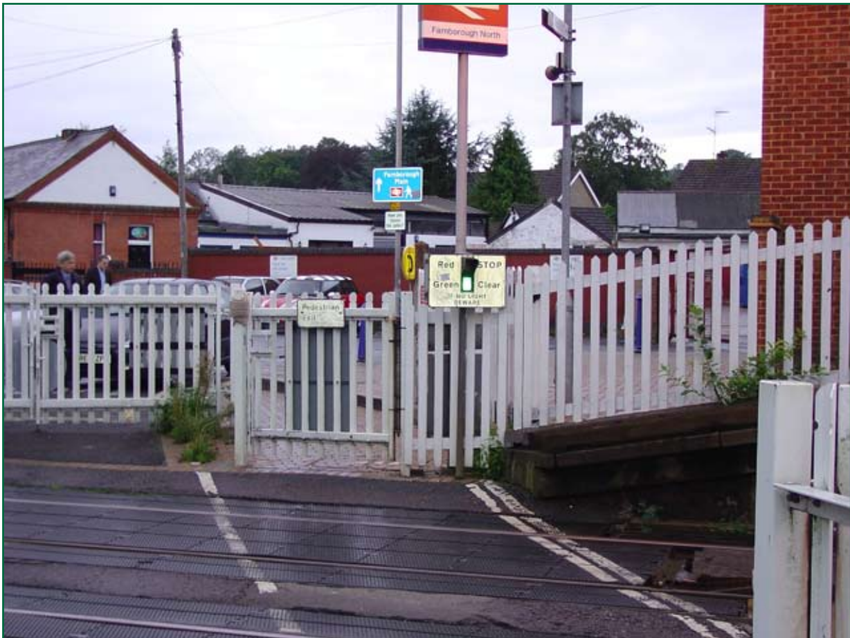
Figure 22: Photograph showing a station pedestrian crossing with miniature stop lights on the far side of the track (in line with current HMRI guidance)
