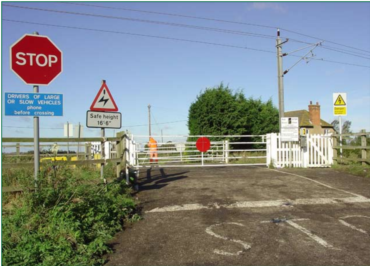
Figure 4: View of crossing approach from East side showing the stop line and gate line
