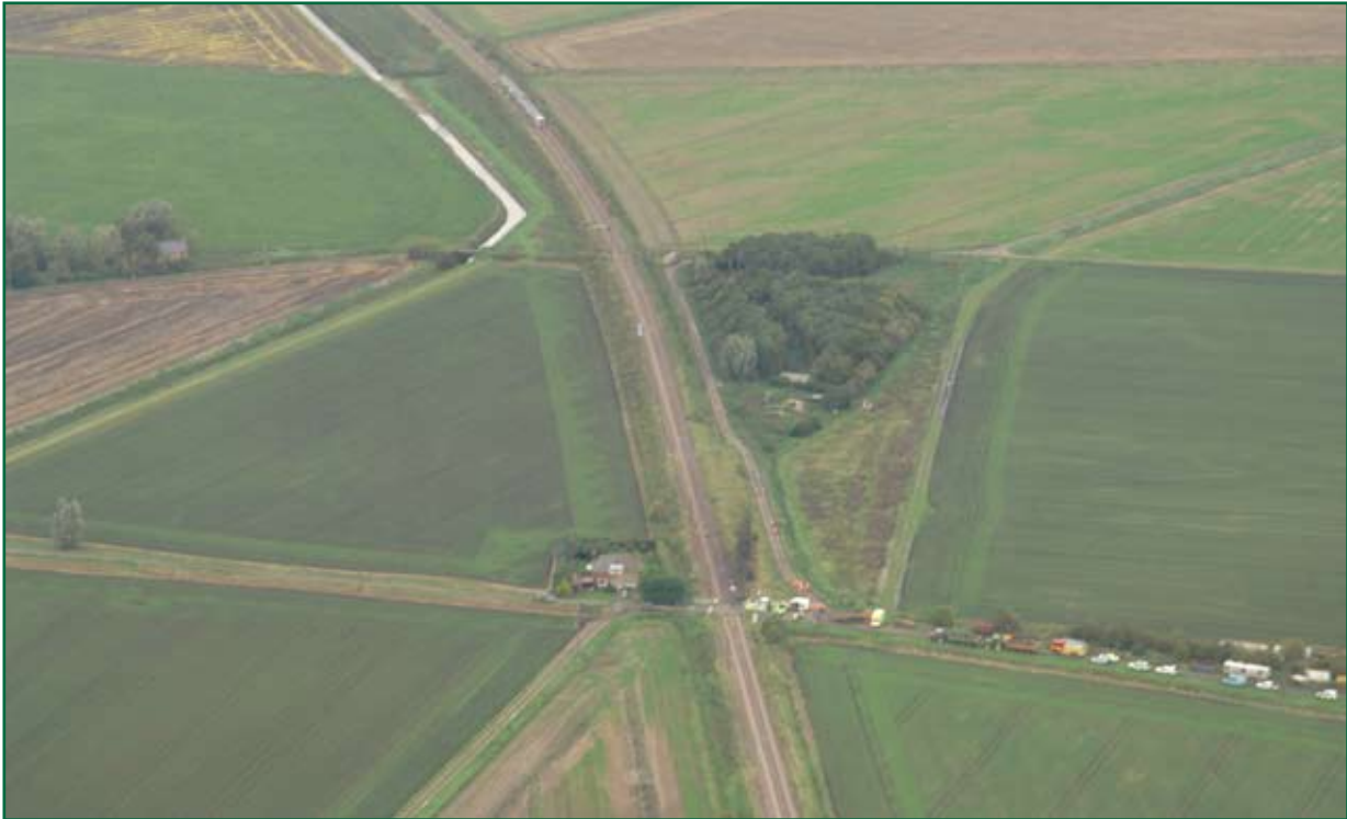
Figure 1: Aerial view of level crossing area
